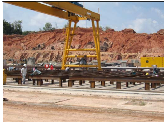
Figure 2: Constructing the pipelay barge
