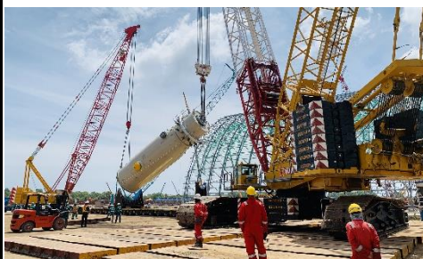
Figure 5: Crawler crane
